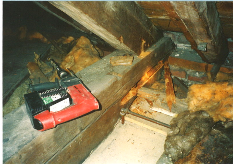
An example of rot in a Tie Beam Bearing End
