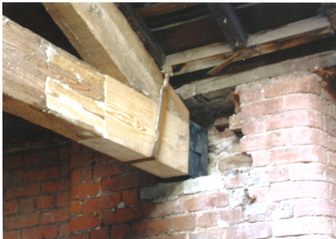
Timber-Resin splice in place
