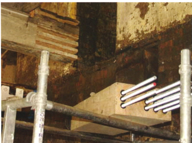
Slots cut, ready to fit Timber Resin Splice
