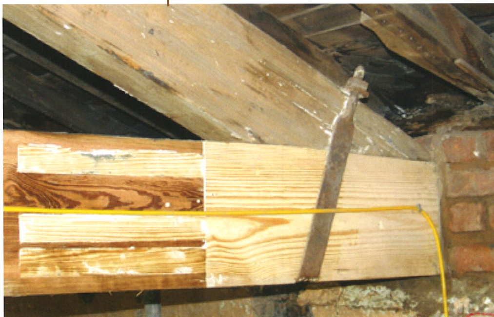
An example of Tie Beam Repair using a Timber Resin Splice, Macintosh Mill. © George Hockey 2007
